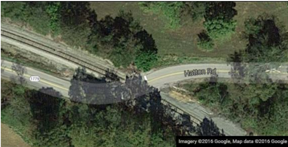
Figure 4.14 Hatton Road crossing.
