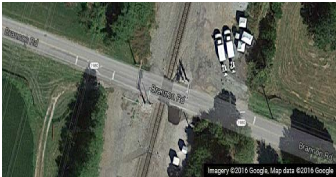
Figure 7.5 Crossing B. Brannon Road crossing (USDOT # 841647U) aerial photo.
