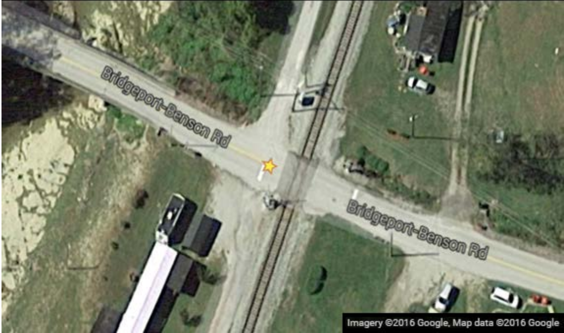
Figure 4.15 Bridgeport-Benson Road crossing.
