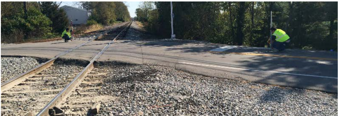
Figure 7.21 Field verification B.
